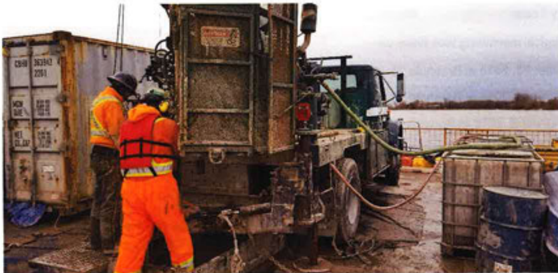
Figure 2: Marathon Underground Drillers and Drill Rig on the Barge.
